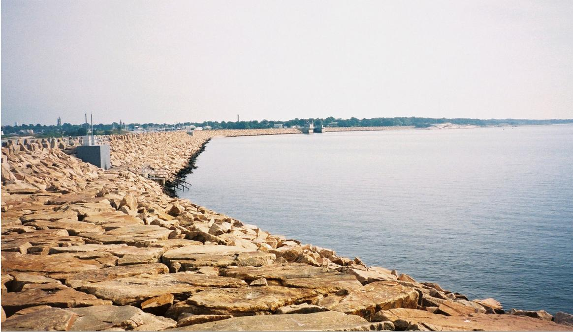
**Figure 20. Hurricane barrier at New Bedford, Massachusetts, looking east toward Fairhaven, showing the open sector gates in the distance and a conduit gate in the foreground.**
