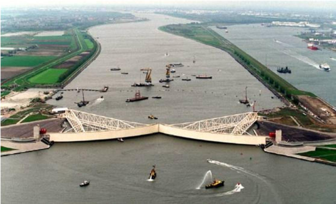
**Figure 24. Stormvloedkering, sector gates which are rotated across the New Waterway in Holland, then sunk to provide the storm surge barrier.**
