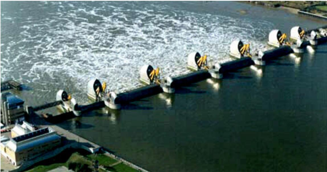
**Figure 22. Thames River tidal barrier with the tainter gates in the undershot position, allowing the river current to scour out any accumulated sediment.**
